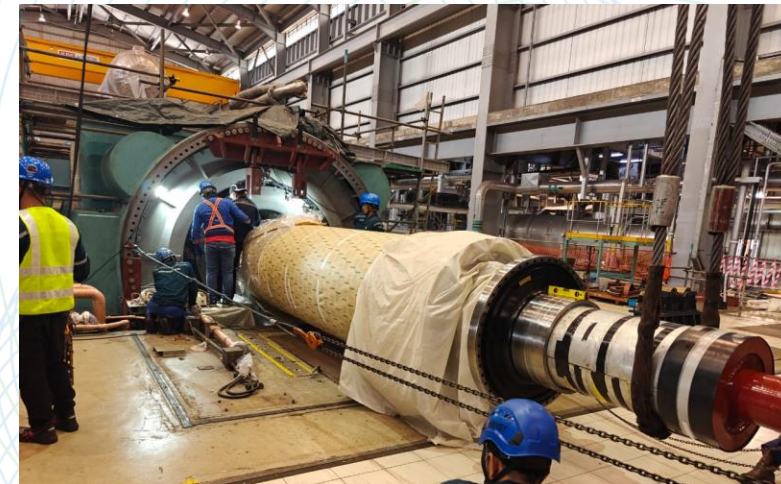
Installation and testing work at TBP – end July
